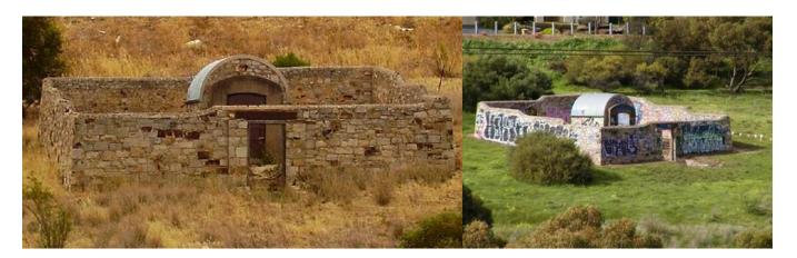
The Yatala Powder Magazine was constructed in 1879 and used to store explosives for the nearby quarry operations. The Magazine had thick stone walls, internal timber lining, perimeter guard walls and a special lightning conductor to protect the sensitive explosives from the risks of sparks and fire. Thick rubber floor mats were used as a precaution and those in charge of handling explosives wore rubber soled shoes.
